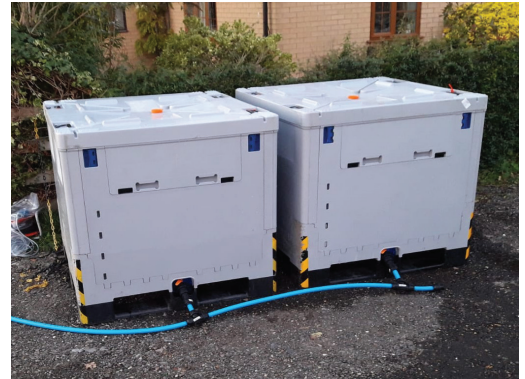
Right: AiS deployment No base, water from the AEWT being pumped directly back into supply.
